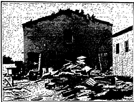
MAIN BUILDING WRECKED BY THE EXPLOSION
